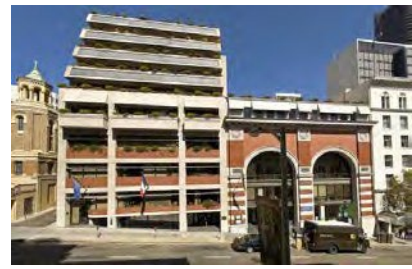
Picture 3 - The Building San Francisco Campus
